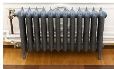
CAST IRON RADIATOR
