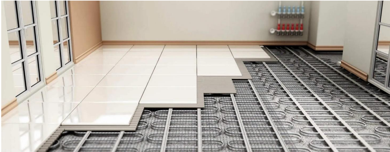
Figure 23. Radiant Floor Heating System
